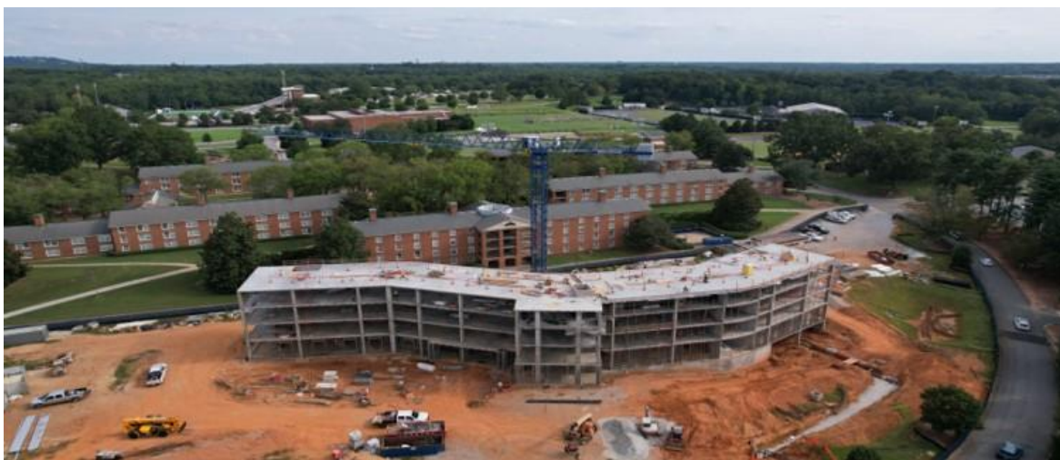
New Freshman Residence Hall under construction
